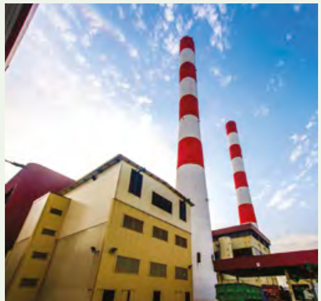
Senoko WTE Plant
