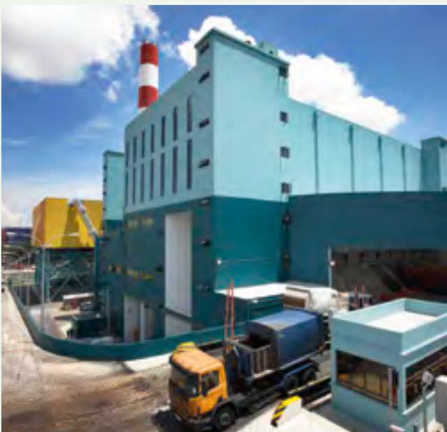
Keppel Seghers Tuas WTE Plant
